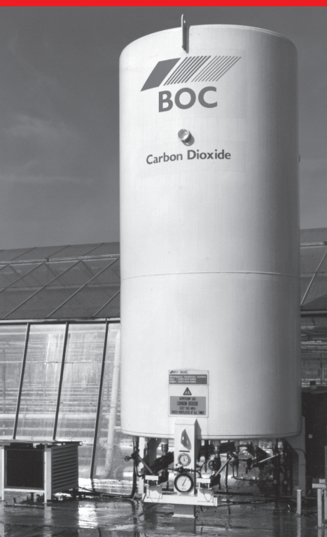
Bulk carbon dioxide installation next to a greenhouse
