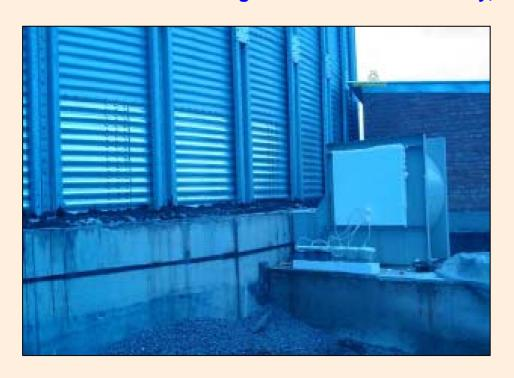
The fumigant gas was applied through tubing to the air duct during the trial period of 5 days
